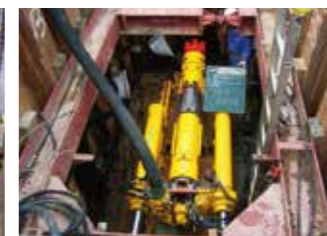
State of jacking (Standard type)
