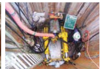
State of jacking (Division starting type)
