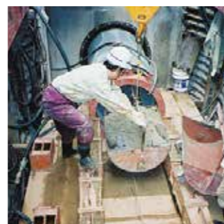
State of underground mucking
