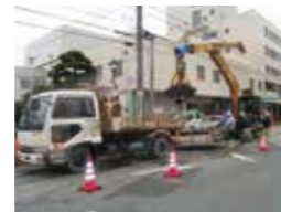
State of excavation
