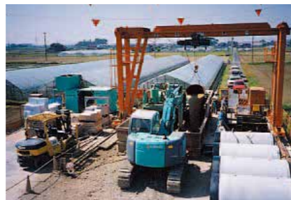
Full view of Construction
