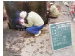
State of welding
