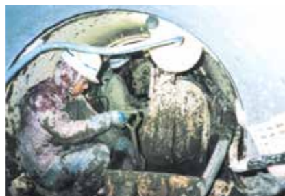
State of inside pipe
