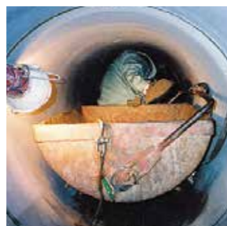
State of pipe excavation
