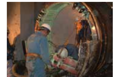
Division and recovery by the excavator
