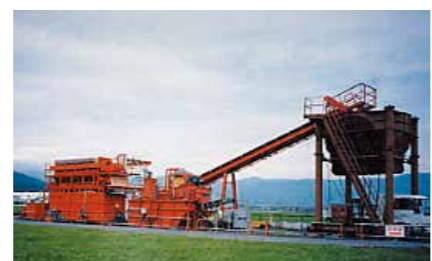
Secondary treatment of slurry
