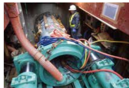
State of shaft
