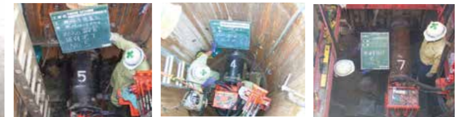
Rotational casing method
