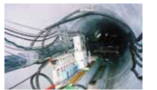
Equipment for middle injection of lubricant
