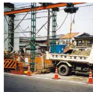
Gantry crane and dump truck on shaft
